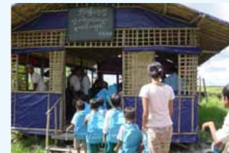
Myanmar: Bamboo TLS built with local materials rapidly after cyclone Nagris.
