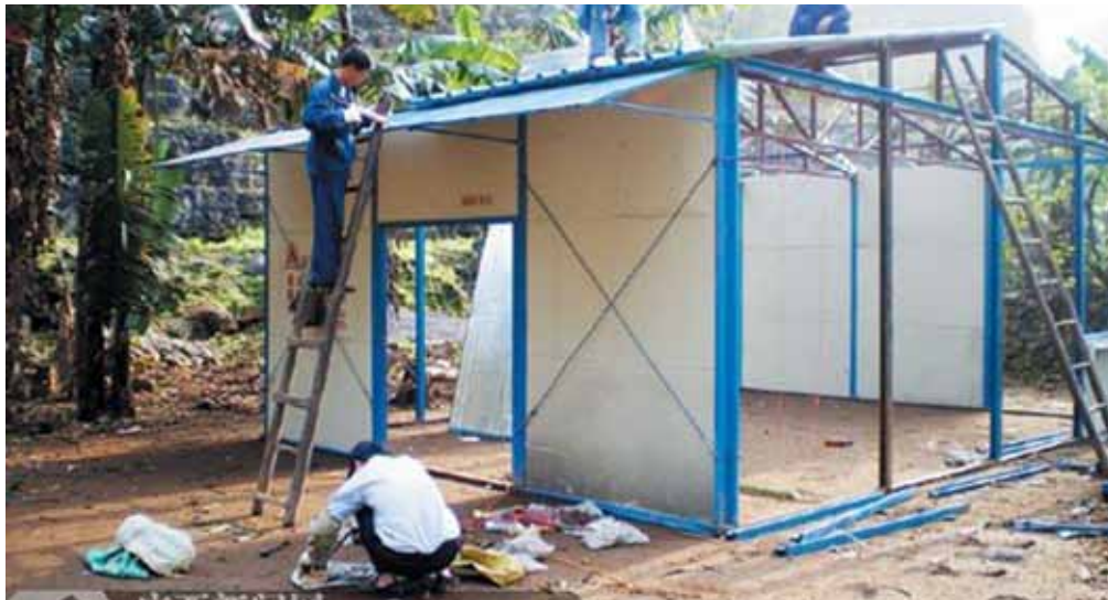
Assembly process of prefabricated classroom
