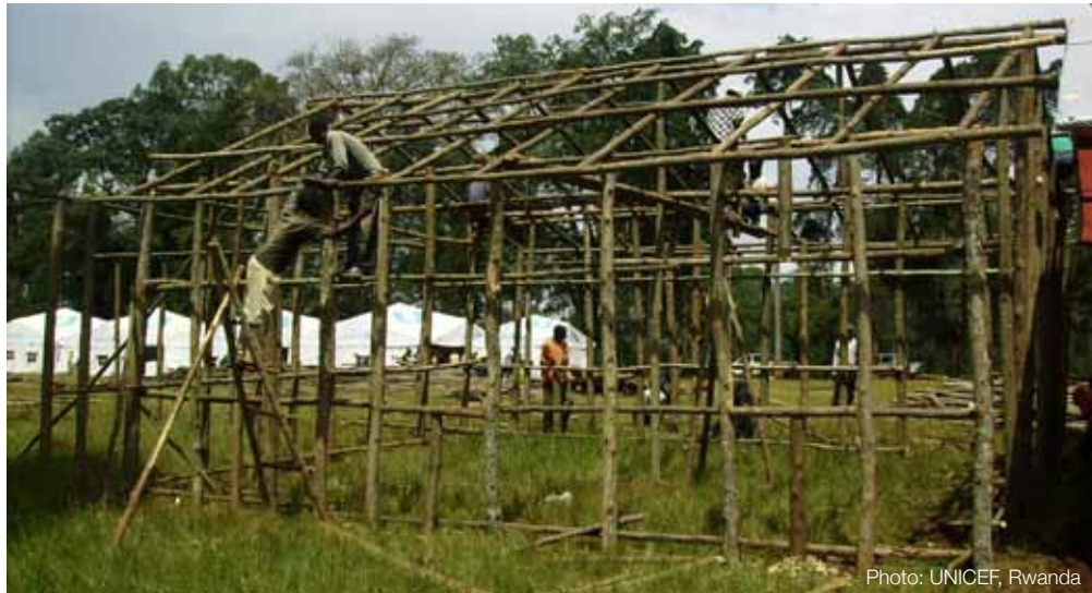
Wooden pole lattice structure, TLS under construction
