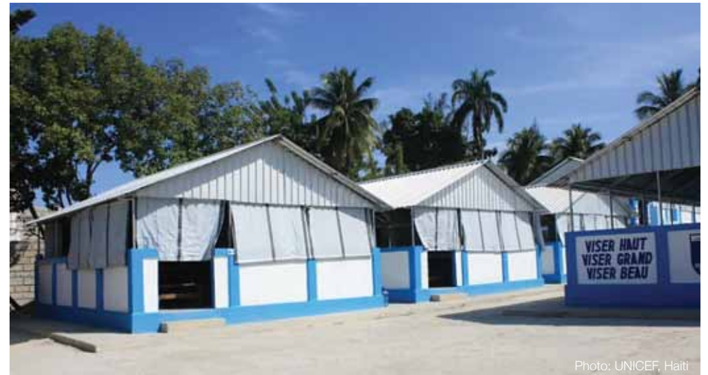
Phase 2, external view of upgraded tent structures
