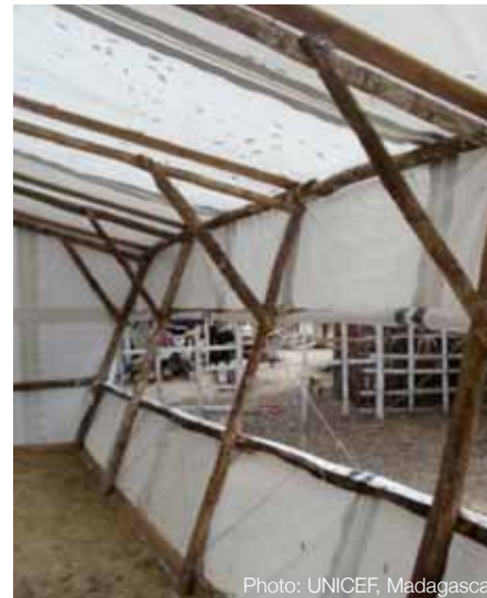
Large openings to guarantee good ventilation
