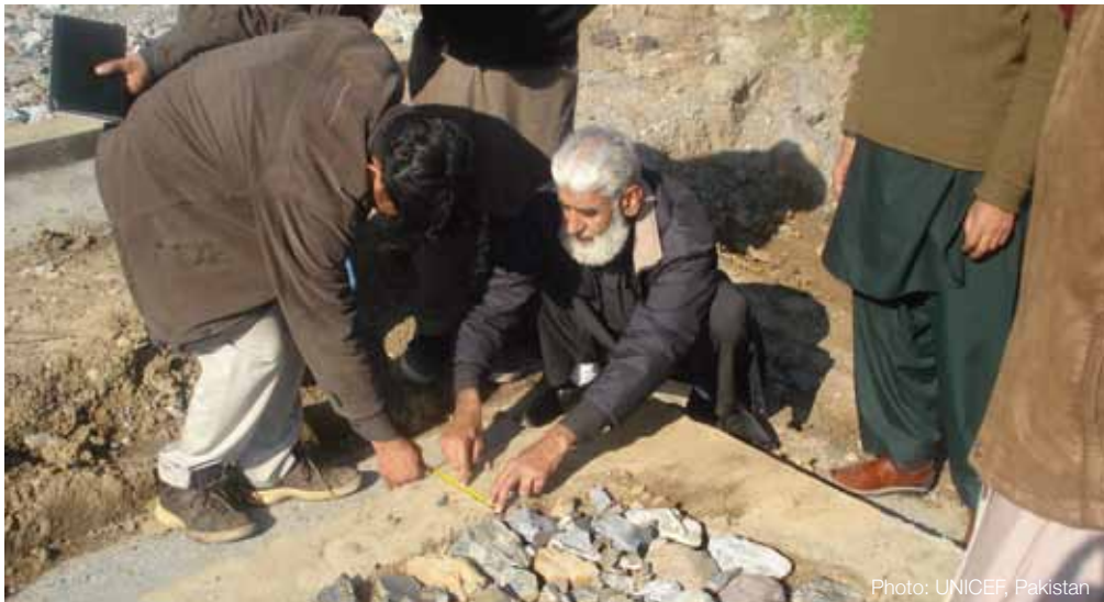
Construction of concrete ring beam
