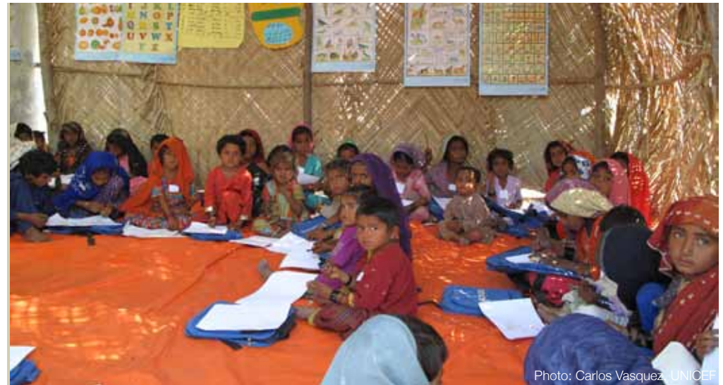
Internal view of bamboo clad structure with tarpaulin floor
