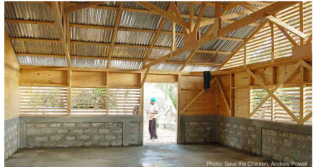
Internal view of masonry/timber TLS version for Ecole Siloe in Jacmel, showing internal natural lighting condition
