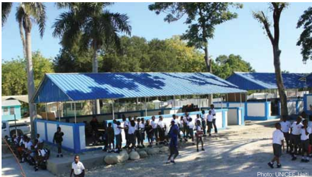
Phase 2, external view of classrooms and school grounds
