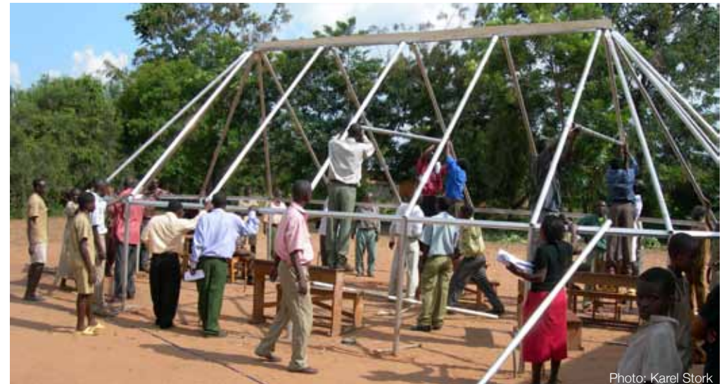
Aluronda tent assembly process
