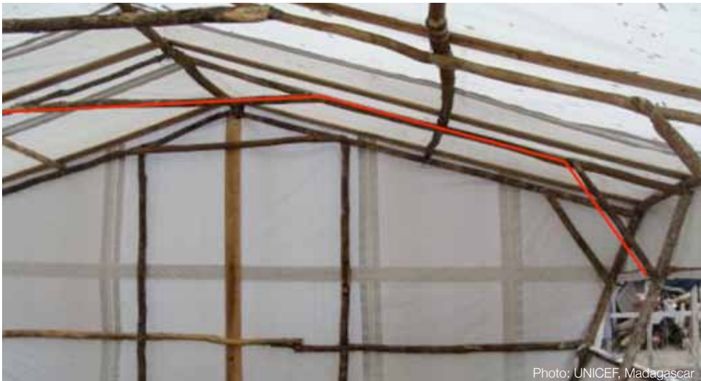
Double layer of tarpaulin can be introduced inside to provide insulation
