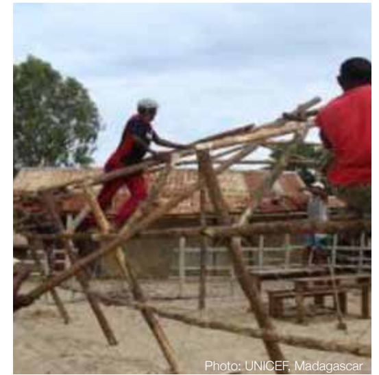
Structure with wooden poles and pegs
