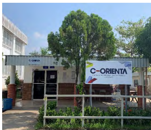
C-Orienta facility in Sonzacate
