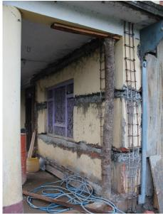
Figure 12. A mason in Bhaktapur drew how they now bent reinforcing steel into foundation footing, rather than simply cutting them at the foundation. The mason explained that he learned this technique as part of his school retrofit training. In North Kathmandu, houses near the school retrofit site were being retrofitted by adding bands and stitches two months after the event. The work was being carried out by local masons who had been trained to retrofit the school. Photo: R. Paci-Green/Risk RED
