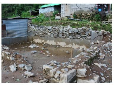
Figure 4. A Ministry of Education template design, which called for vertical rebar to be placed in stone walls, completely collapsed in every block assessed with this design. While now removed, after the earthquake, the classrooms were filled with stone from the collapsed walls. Photo: R. Paci-Green/Risk RED
