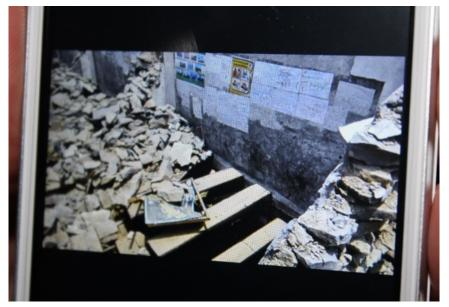
Figure 10. In Rasuwa, a poorly retrofitted stone school collapsed. Photos from the principal attest to the fact that few students would have been able to evacuate or survive the collapse.
