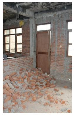
Figure 2. School building 101-1, which experienced only moderate shaking in Bhaktapur, was deemed unsafe for school use because unreinforced partition walls separated from the reinforced concrete frame and became unstable. Damage to unreinforced partition or infill walls can injure or kill students and block exits. The safety of these walls is routinely ignored by engineers and communities alike. Photo: R. Paci-Green/Risk RED
